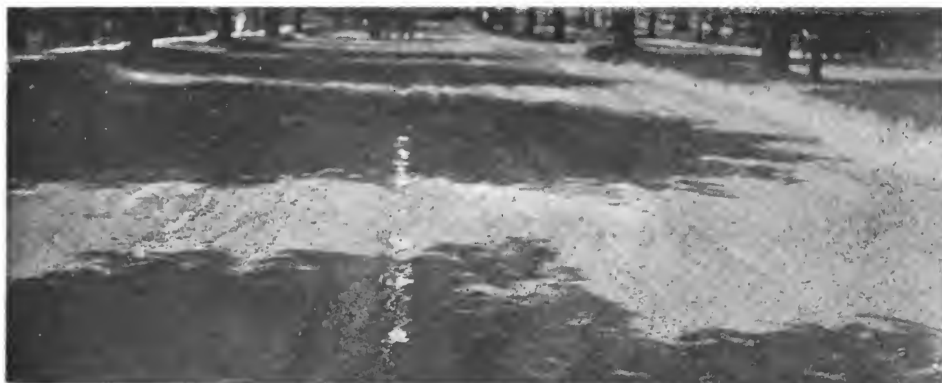
Striking Illustration of Damage Done by Horses and Narrow Tires on a New York Driveway.
